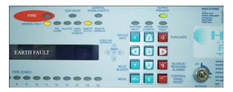
A – This indicates that one of the external cable circuits has either the positive or negative cores touching down to the building earth usually via the cable earth core, this must be rectified by a competent person before fault will clear.
