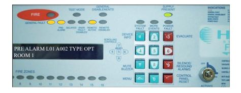
A - This indicates that a detector has recorded a higher than normal analogue value which could signal an impending fire condition or detector requires cleaning.
