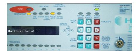
A – Panel is indicating a fault on the internal power supply unit (PSU), power supply is indicating a high impedance fault between the charger output and batteries. Check condition of battery terminals and leads, check for loose or poor fitting battery connectors. May also indicate a fault with the power supply unit.
